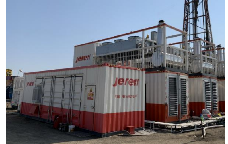
1MW/1.2MWh Oil Rig BESS
