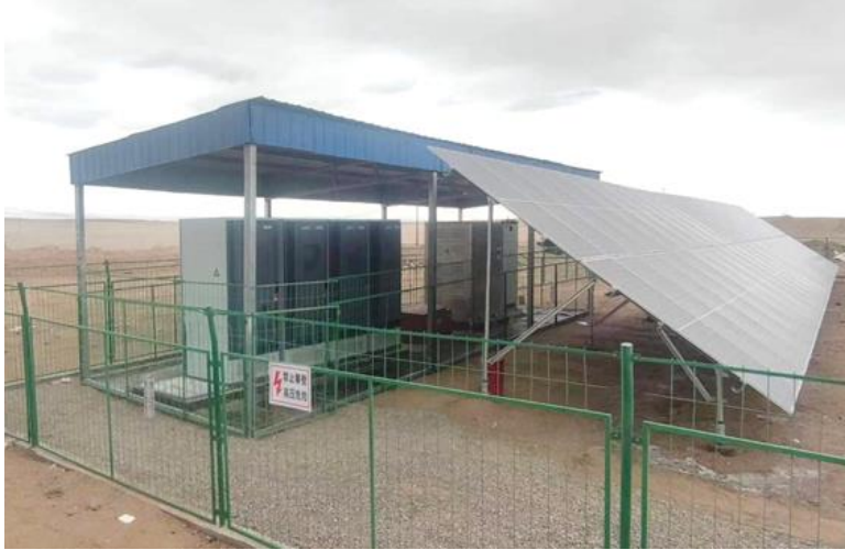
0.3MW/0.64MWh Salt Mine BESS
