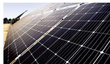
JINERGY experimental power project
